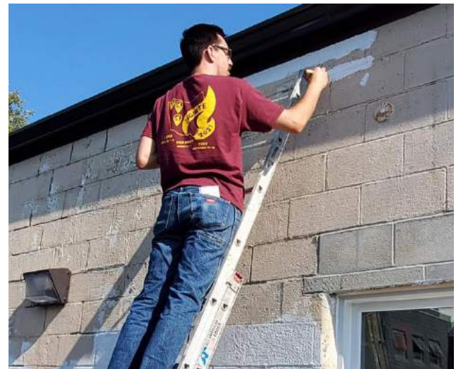
An IGNITE volunteer giving a building a fresh coat of paint
